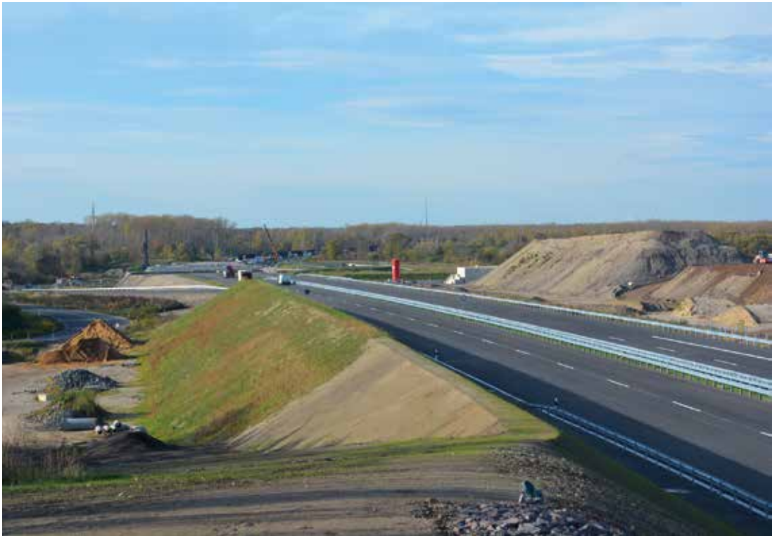
Completion of the section of the A 72 Chemnitz-Leipzig motorway near Rötha, Leipzig district
