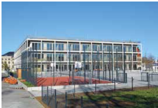
Construction of a new secondary school at Hartmannplatz in Chemnitz.
