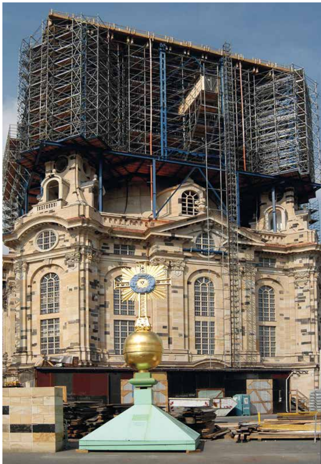
Dresden Frauenkirche during reconstruction, 1995
