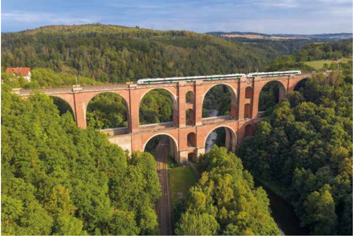
Elster Valley Bridge, Vogtland district
