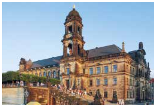
The Dresden Ständehaus, one of the most distinctive buildings in Dresden's Old Town (built 1901-1907), served as the seat of the Saxon Landtag during the Weimar Republic from 1919 to 1933. Its final session on 21 February 1933 marked the temporary end of democracy in Saxony.
