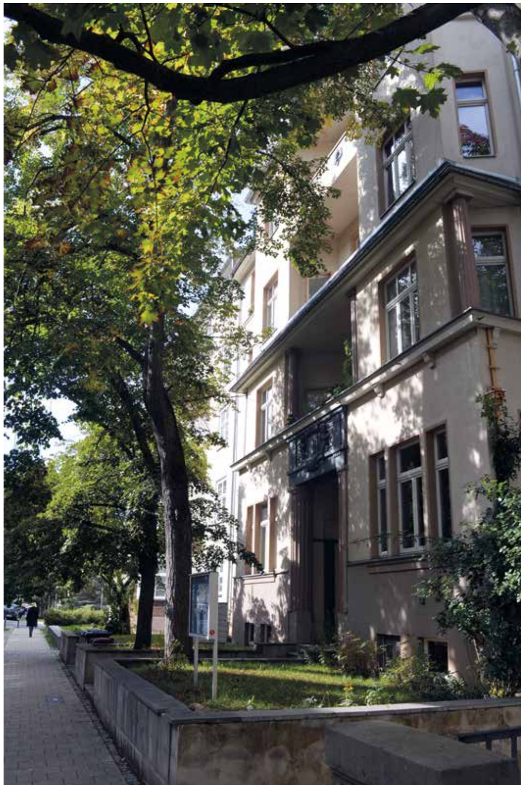
Chemnitz-Kaßberg, Wilhelminian-era building
